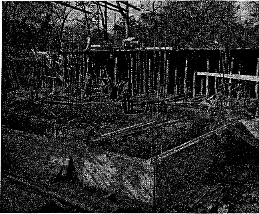
The library foundation as it looked on November 3.
