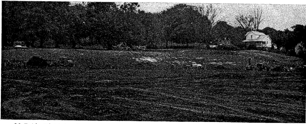
McBride Field in August, when grading was still going on.
